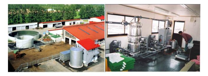
**Fig. 3** Thermophilic biogas plant (4 tons per a day) and bench scale ammonia stripping plant attached to the biogas plant in Obihiro University of Agriculture and Veterinary Medicine
